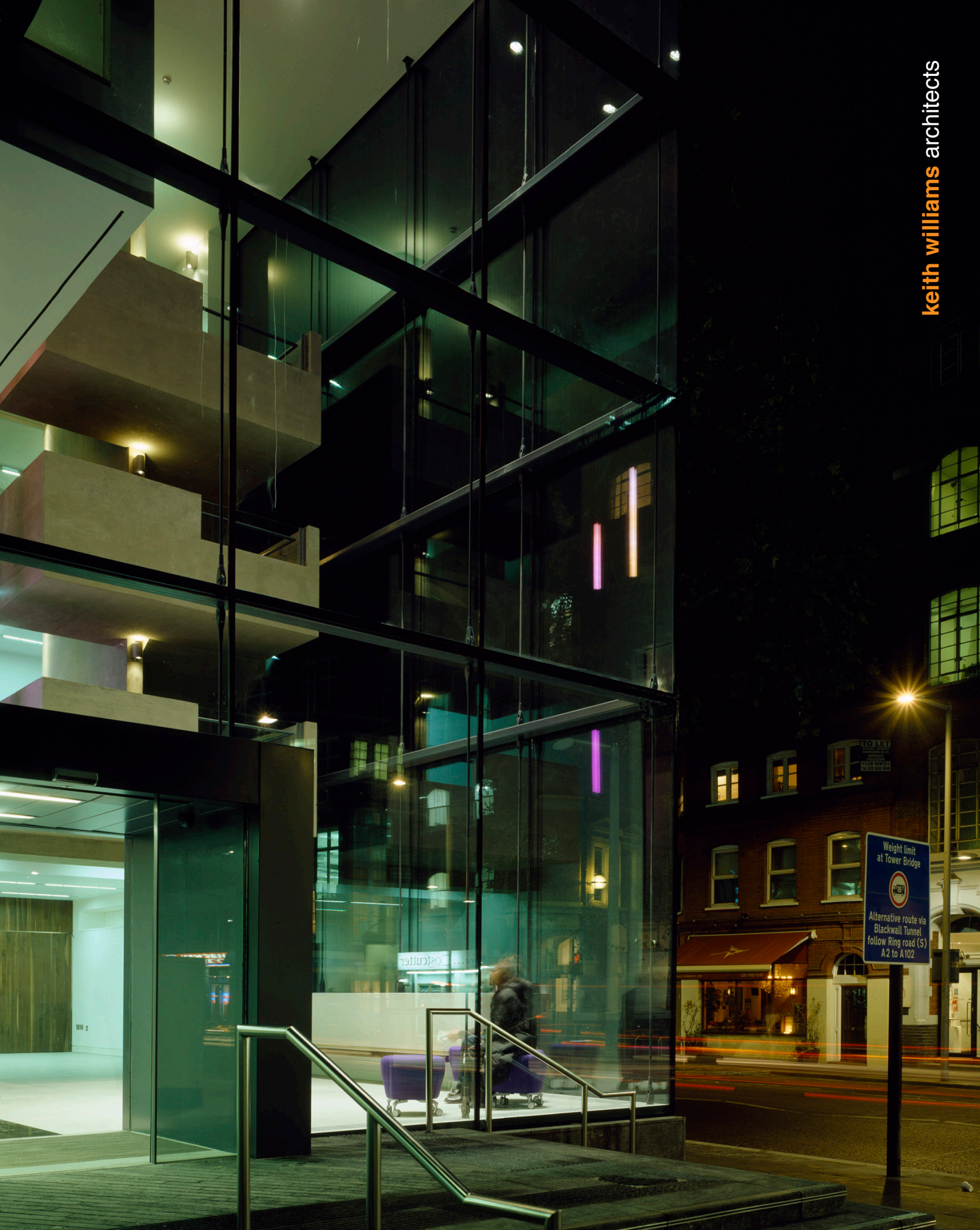
main foyer with cascading stair to the Weston Theatre 7m above the street
